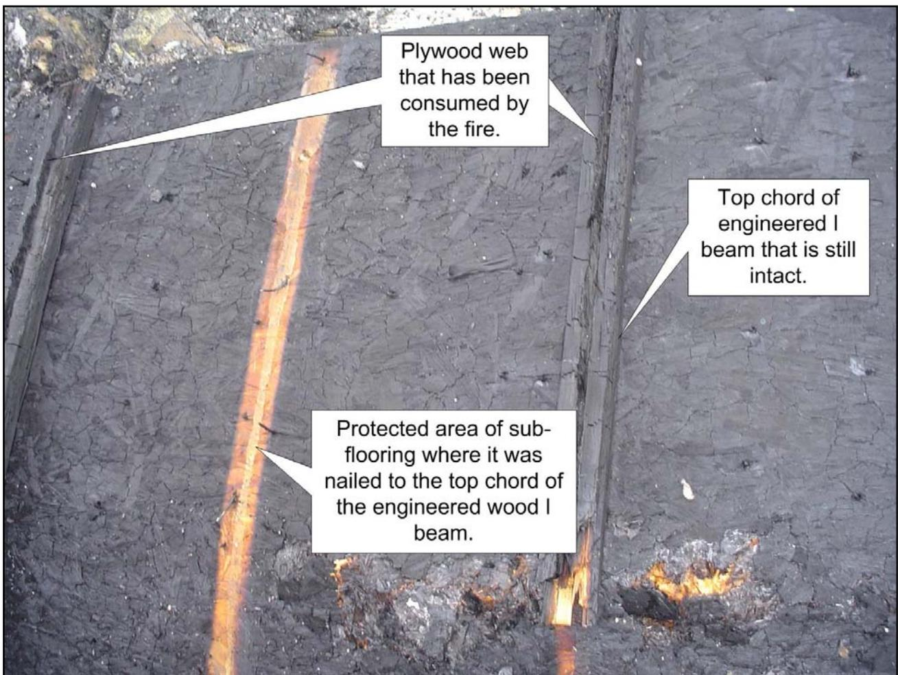
**Photo 2. Engineered Wood I-Beam Webs Consumed by Fire**
