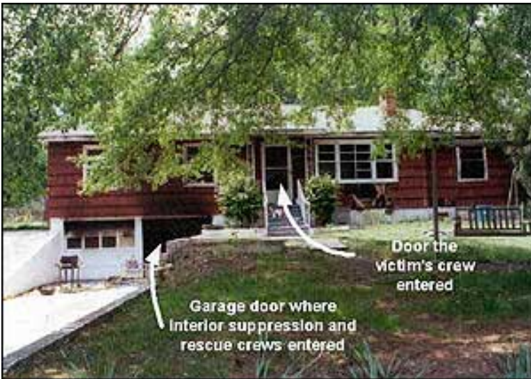
NIOSH F2000-26 - Firefighters made an aggressive interior attack across the first floor, over the involved basement, at this residence. As the crew advanced to the rear of the home, in zero visibility and hot conditions, the victim died after falling through the fire weakened floor.
